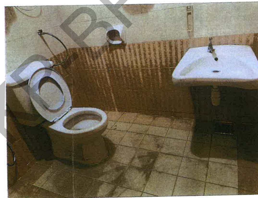
Existing site picture for references
