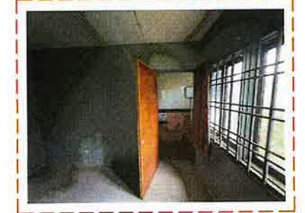
SERVANT ROOM + TOILET 1
